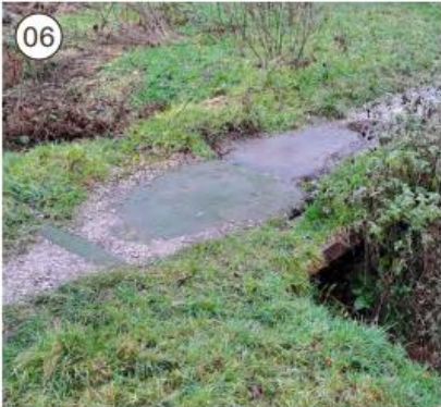
BRIDGE ACROSS WESTERN DITCHLINE
